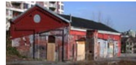
Gas Works Heritage Building can be adapted as a public building to support a variety of new community programs
